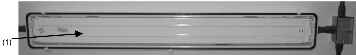
Figure 4-41. Ceiling light with metal cover exposed.
