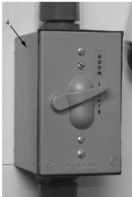
Figure 5-11. Group 0110, Door Entry Wall (Inside)
