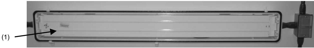
Figure 4-9. Ceiling light with bulbs removed.
